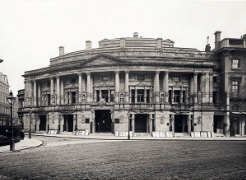
King Edward Memorial and Victoria Rooms, Bristol.
